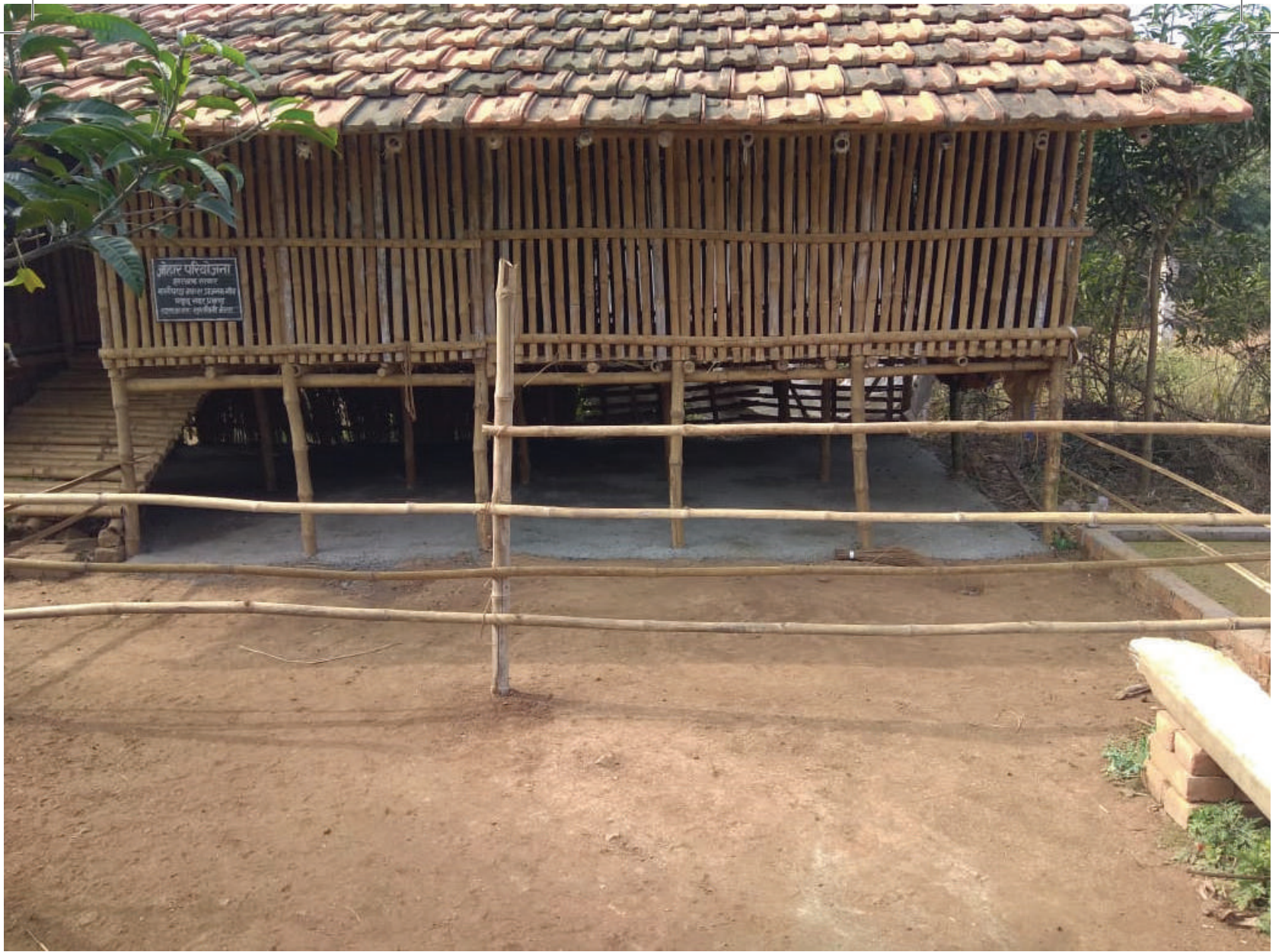
Figure 7- Low-cost Goat Shed Constructed with Bamboo
